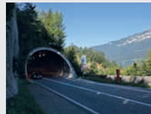
D Sengg tunnel
